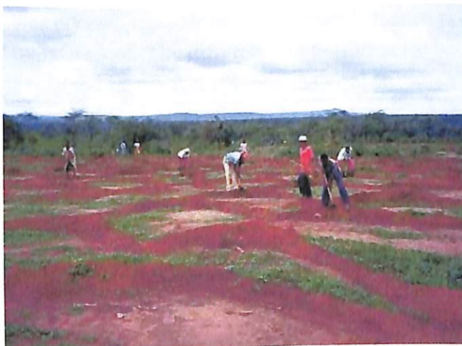
Catchment construction (W-shaped)
